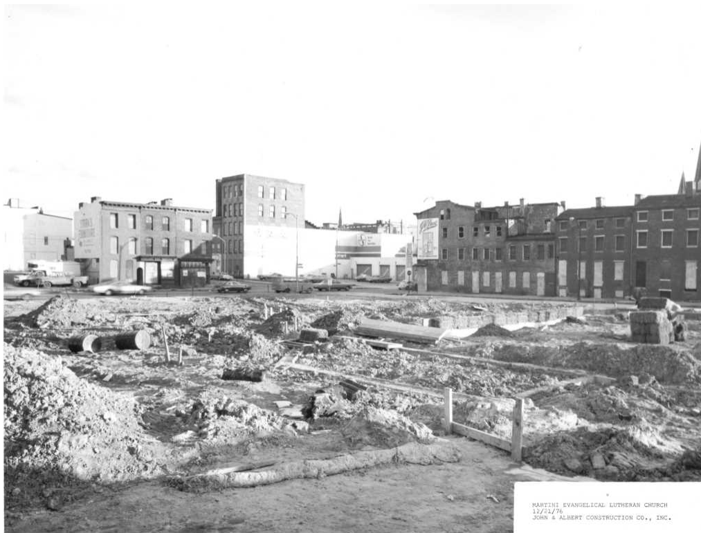
Construction Site for the New Martini
